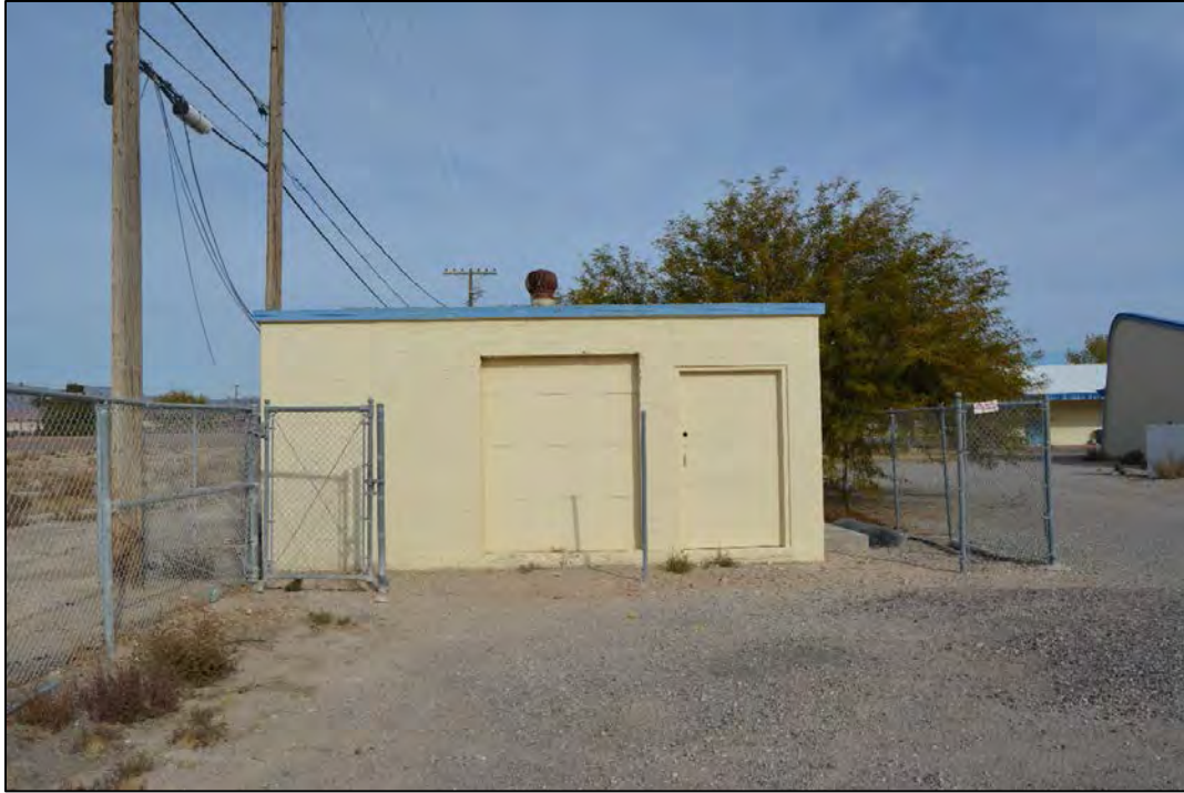
Figure 114. Unnumbered structure, looking north.
