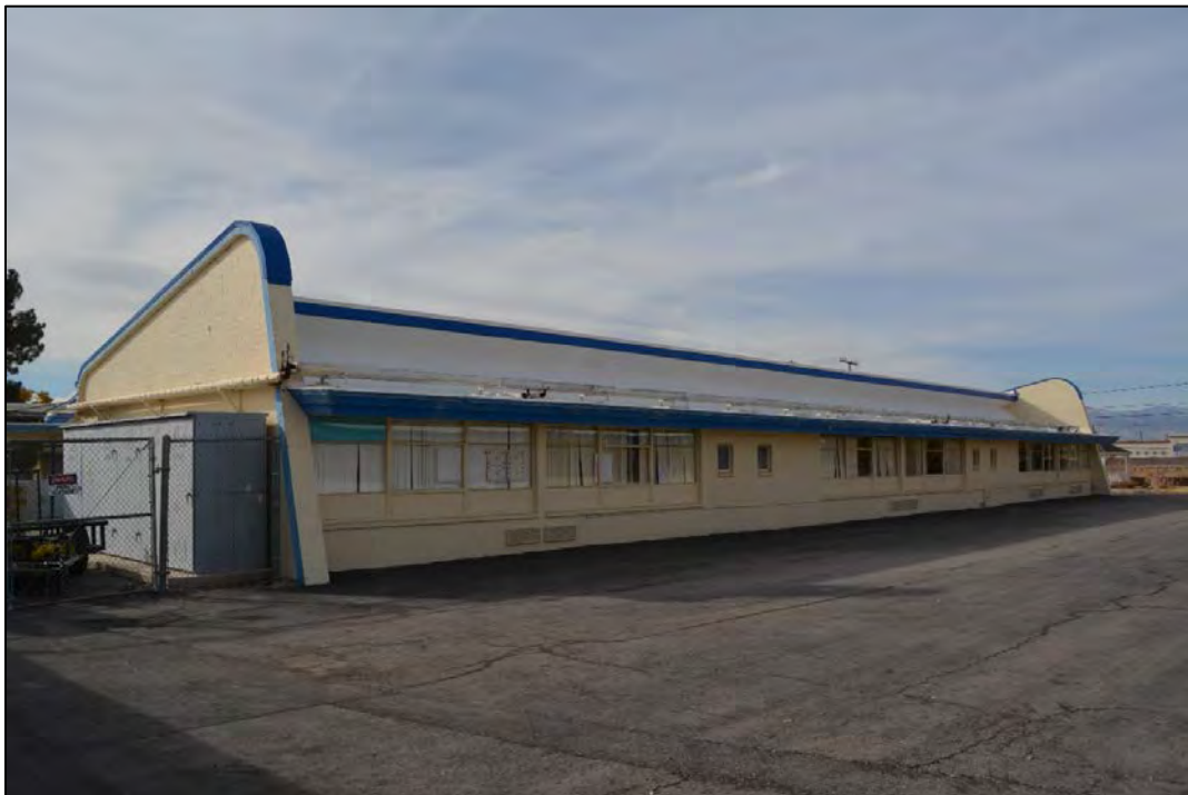
Figure 83. Facility 1789 east and north elevations, looking southwest.
