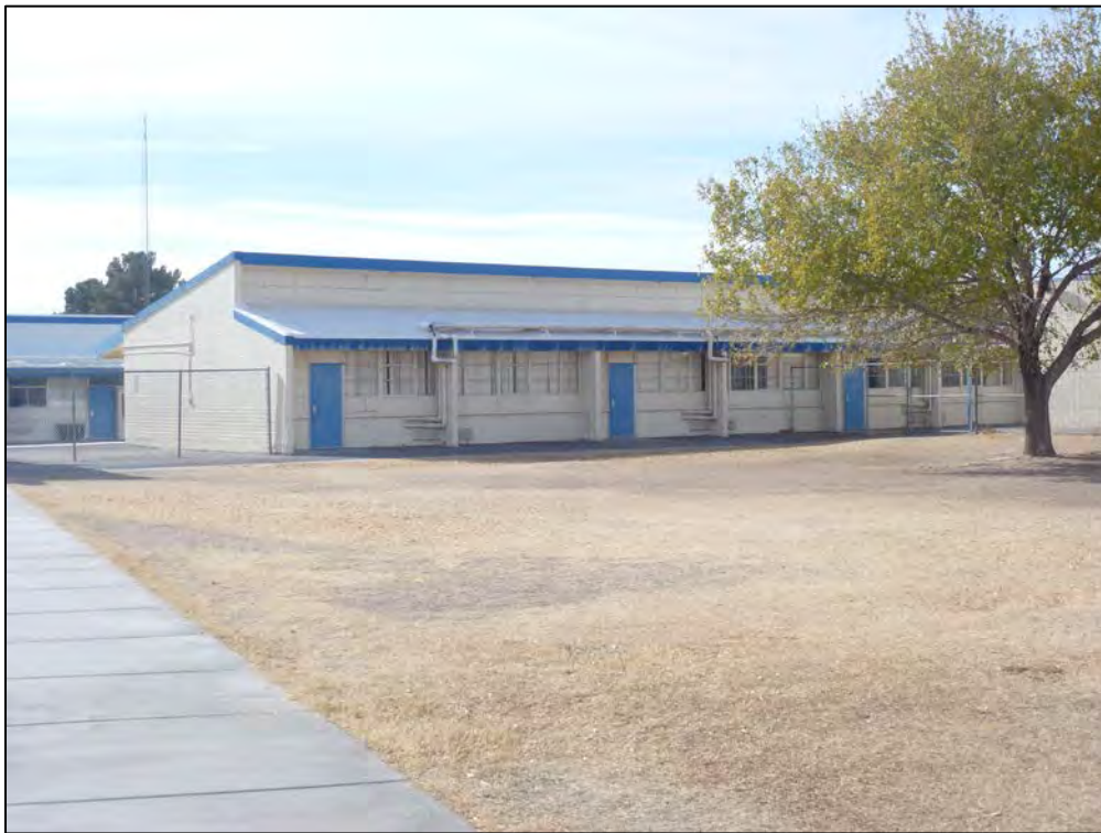
Figure 66. Facility 1785 north elevation, looking southwest. Note: Roof windows filled.
