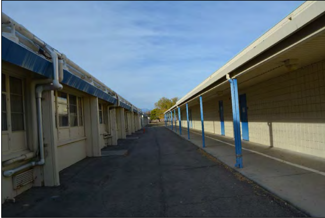
Figure 76. Courtyard between Facility 1785 (left) and 1787 (right), looking northwest.
