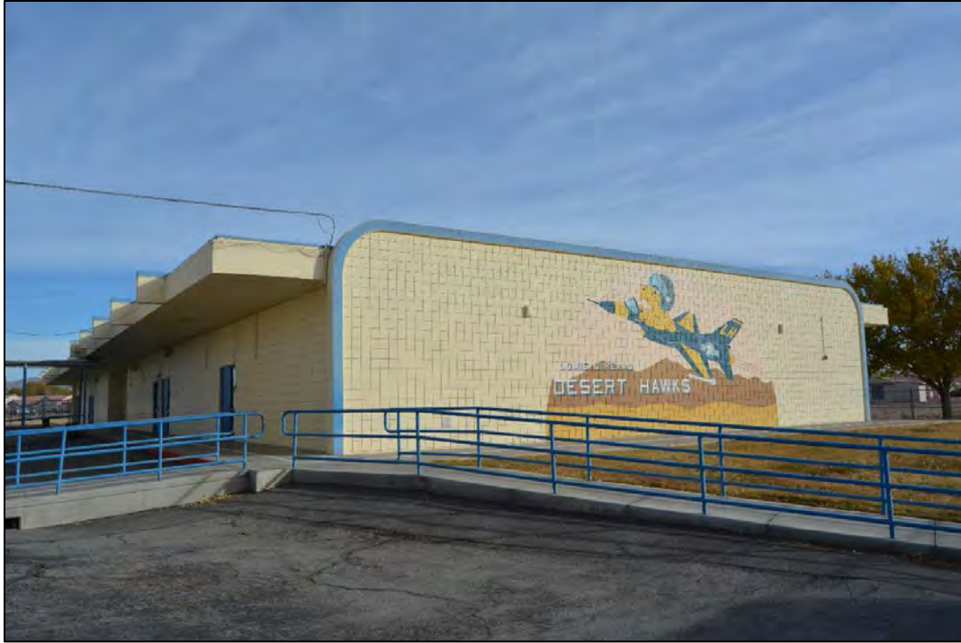
Figure 67. Facility 1786 south elevation, looking north.
