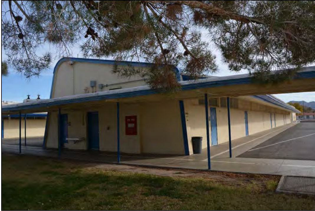
Figure 52. Facility 1783 west and south elevations, looking northeast.
