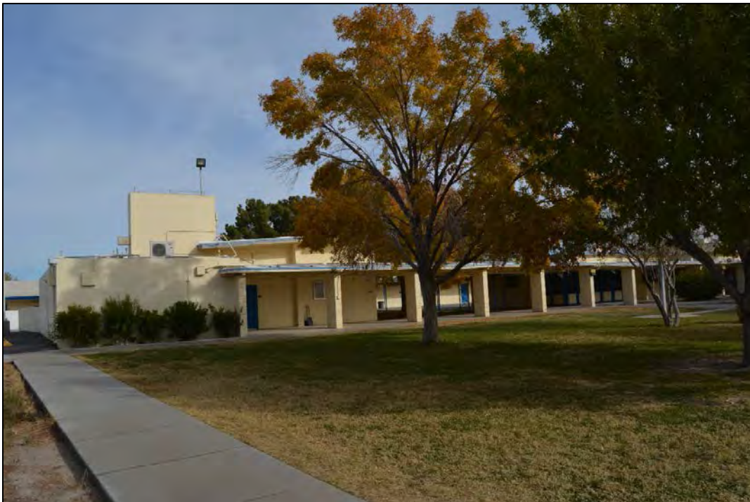
Figure 112. Sidewalk leading to Facility 1790, looking north.
