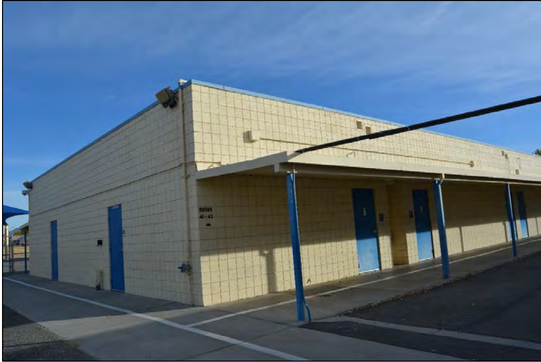
Figure 72. Facility 1787 west and south elevations, looking northeast.
