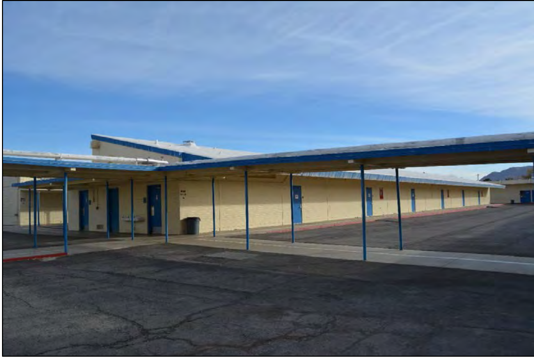
Figure 61. Facility 1785 west and south elevations, looking northeast.
