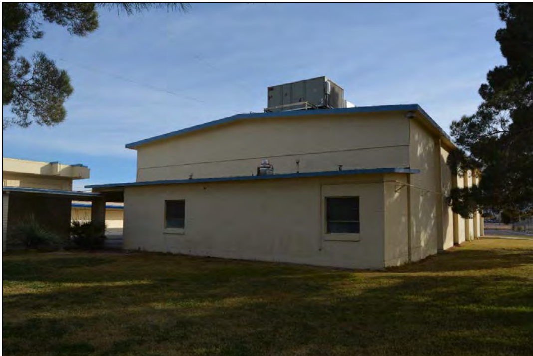
Figure 48. Facility 1782 west elevation, looking east. Note: One-story wing spanning the west elevation.
