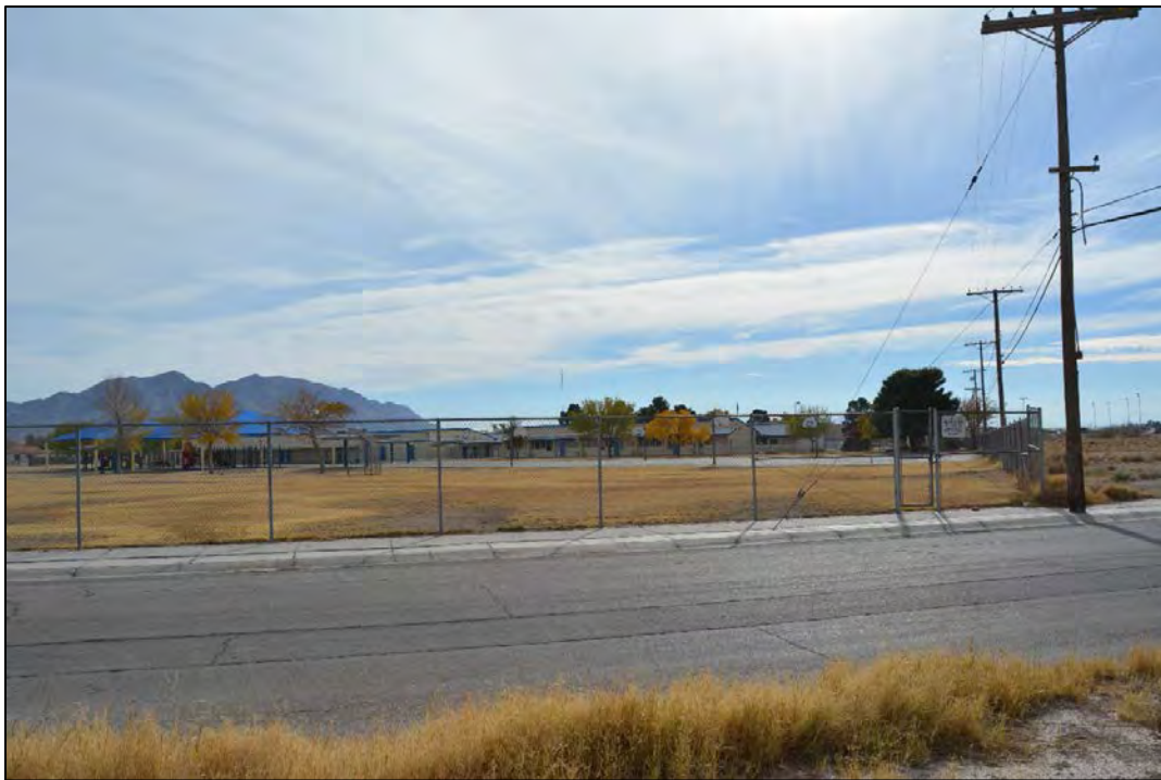
Figure 96. Chain-link fence at the northwest campus boundary, looking south.
