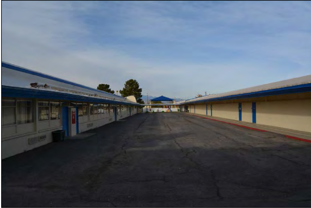
Figure 60. Courtyard between Facility 1783 (left) and Facility 1784 (right), looking west.
