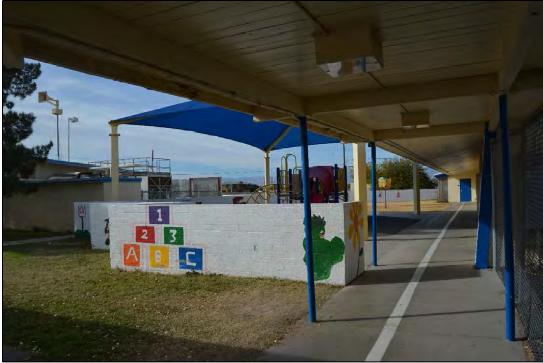
Figure 113. View of covered sidewalk located adjacent to Facility 1789, looking west.
