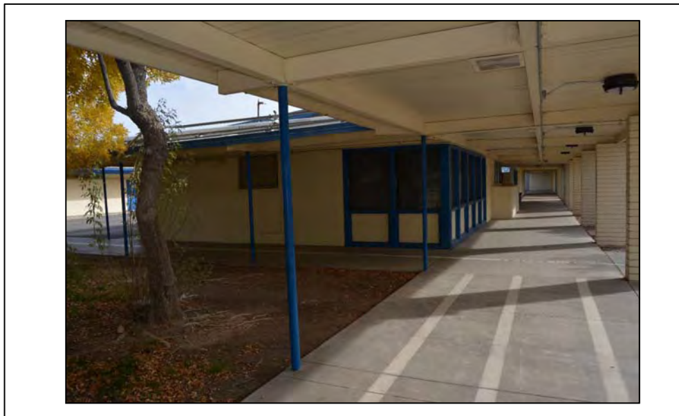
Façade: West Facing: E Photographer: Serra Akboy-İlk Date: 12/11/16
