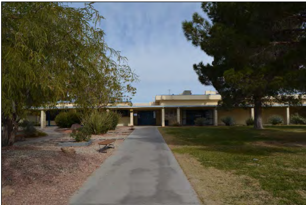
Figure 38. Facility 1781 south elevation, looking north.
