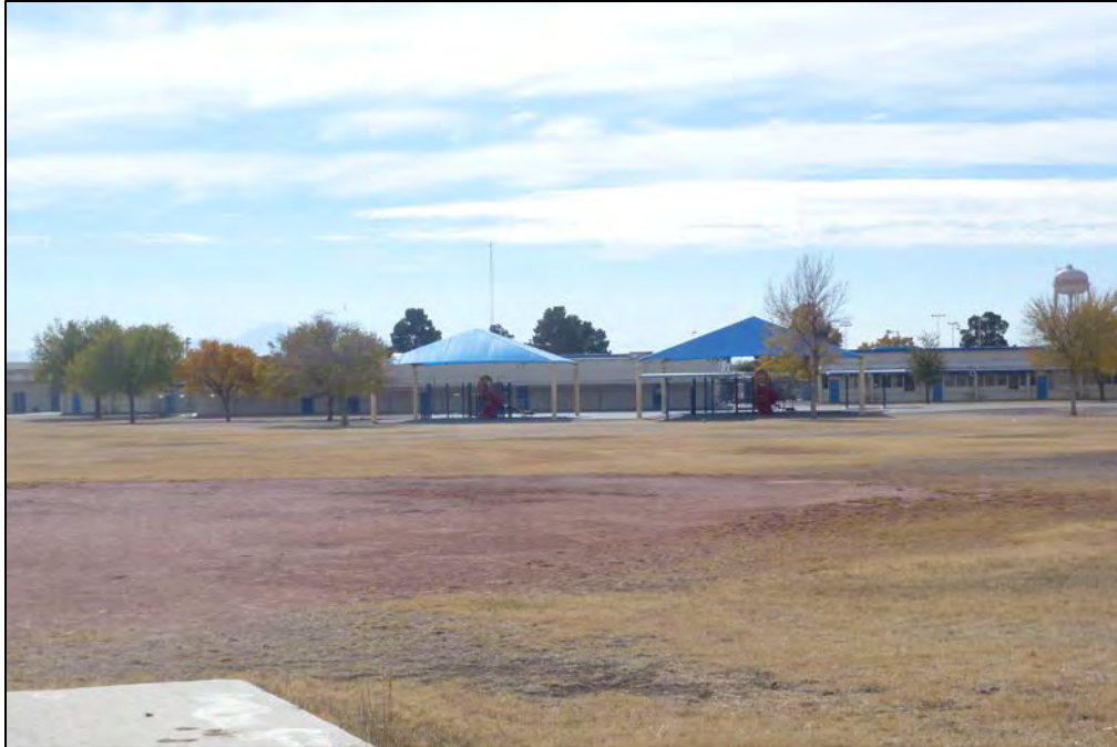
Figure 105. Two overhead protections located in the main playground, looking south.
