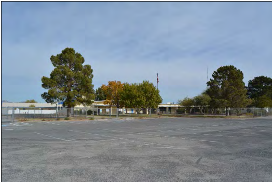
Figure 109. Main parking lot, looking north. Facilities 1789, 1790, and 1781 (left to right) are seen in the background.
