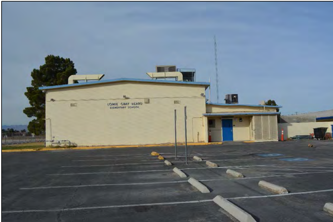
Figure 50. Facility 1782 east elevation, looking west. The parking lot (Facility 50000) is on the front.
