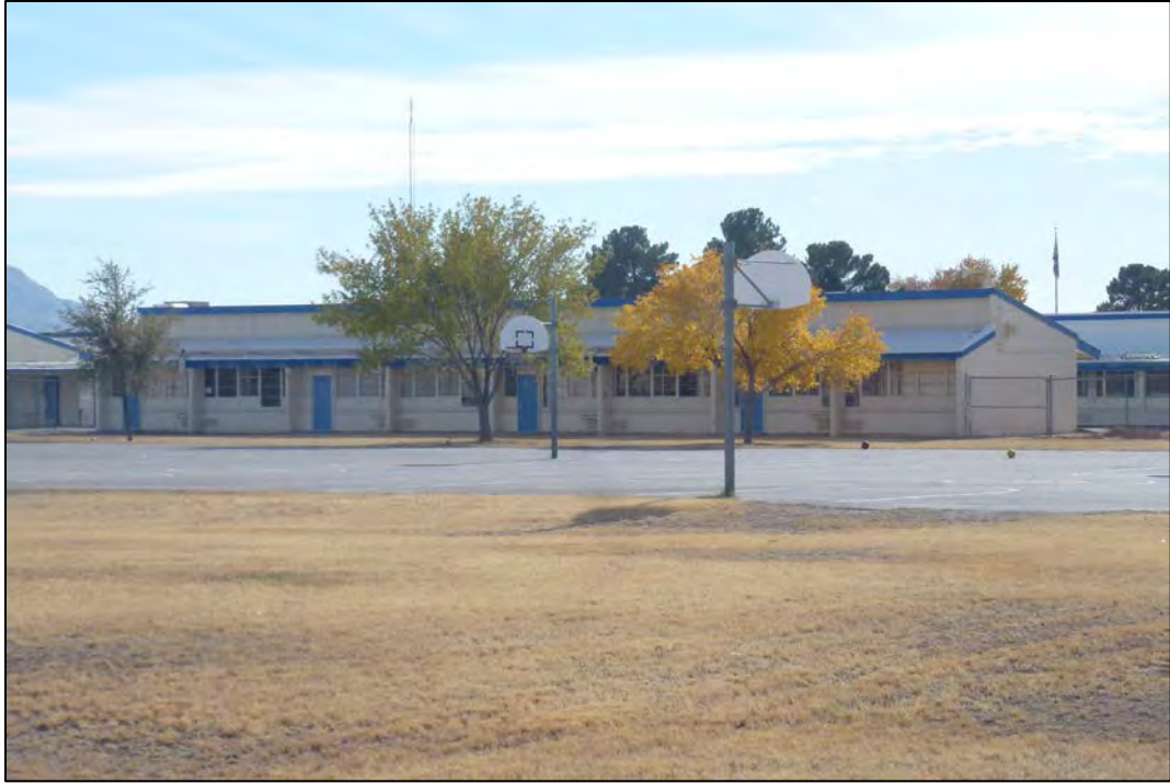
Figure 77. Facility 1788 north and west elevations, looking southeast.
