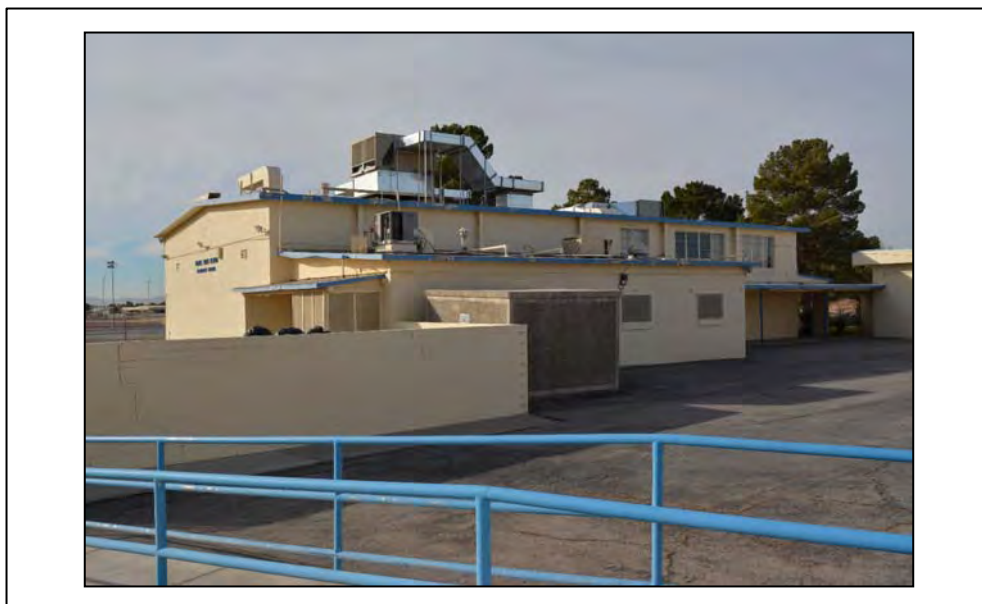
Façade: East and North Facing: SW Photographer: Serra Akboy-İlk Date: 12/11/16
