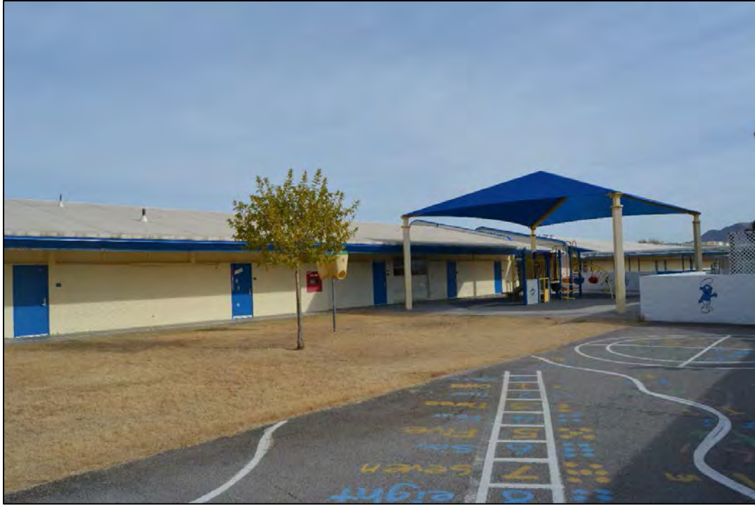
Figure 88. Facility 1789 south elevation and adjacent enclosed courtyard and playground, looking northeast.
