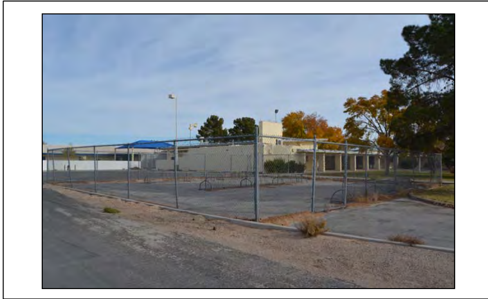
Façade: N/A Facing: NE Photographer: Serra Akboy-İlk Date: 12/11/16
