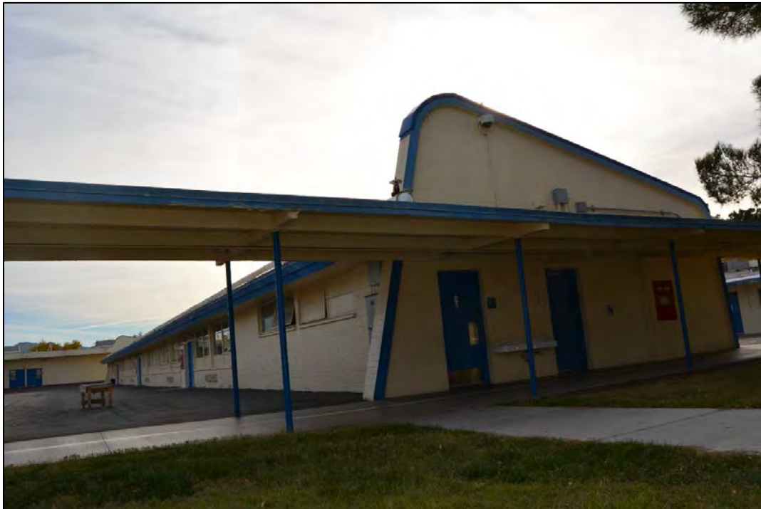
Figure 53. Facility 1783 west and north elevations, looking southeast.
