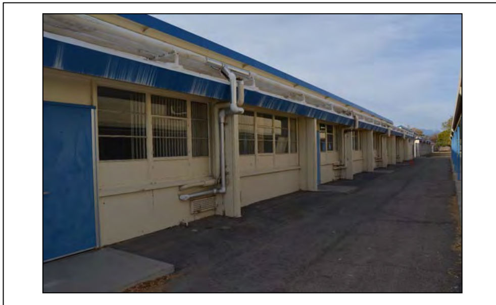
Façade: North Facing: SW Photographer: Serra Akboy-İlk Date: 12/11/16
