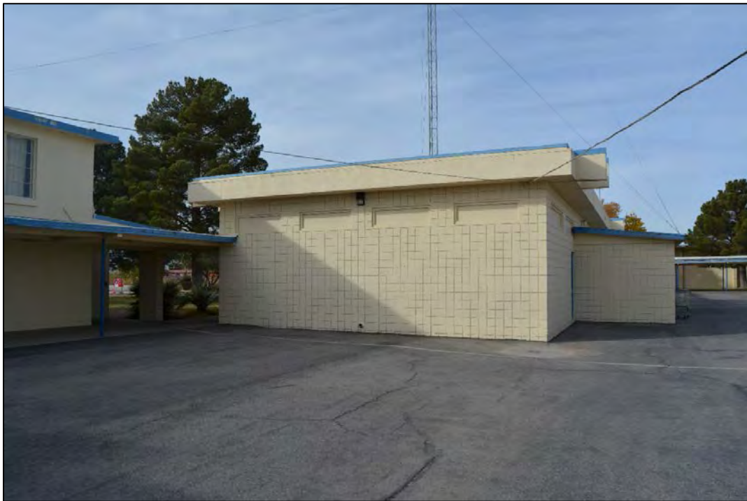
Figure 40. Facility 1781 east elevation, looking west. Note: Facility 1782 is seen on the left.
