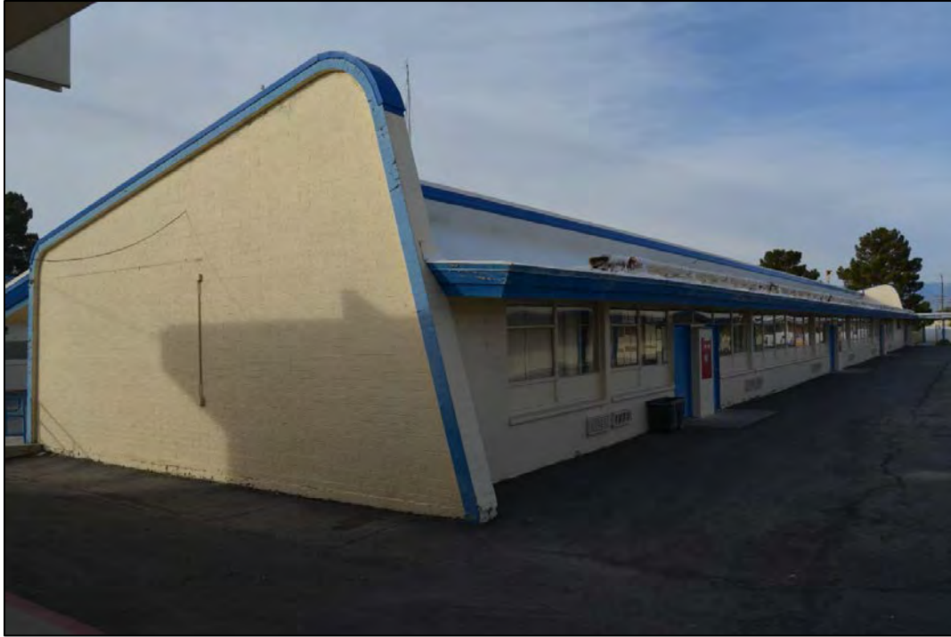
Figure 56. Facility 1784 east and north elevations, looking southwest.
