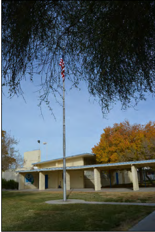
Figure 95. View of the flagpole (Facility 3200), looking north. Note: Facility 1790 is on the background.
