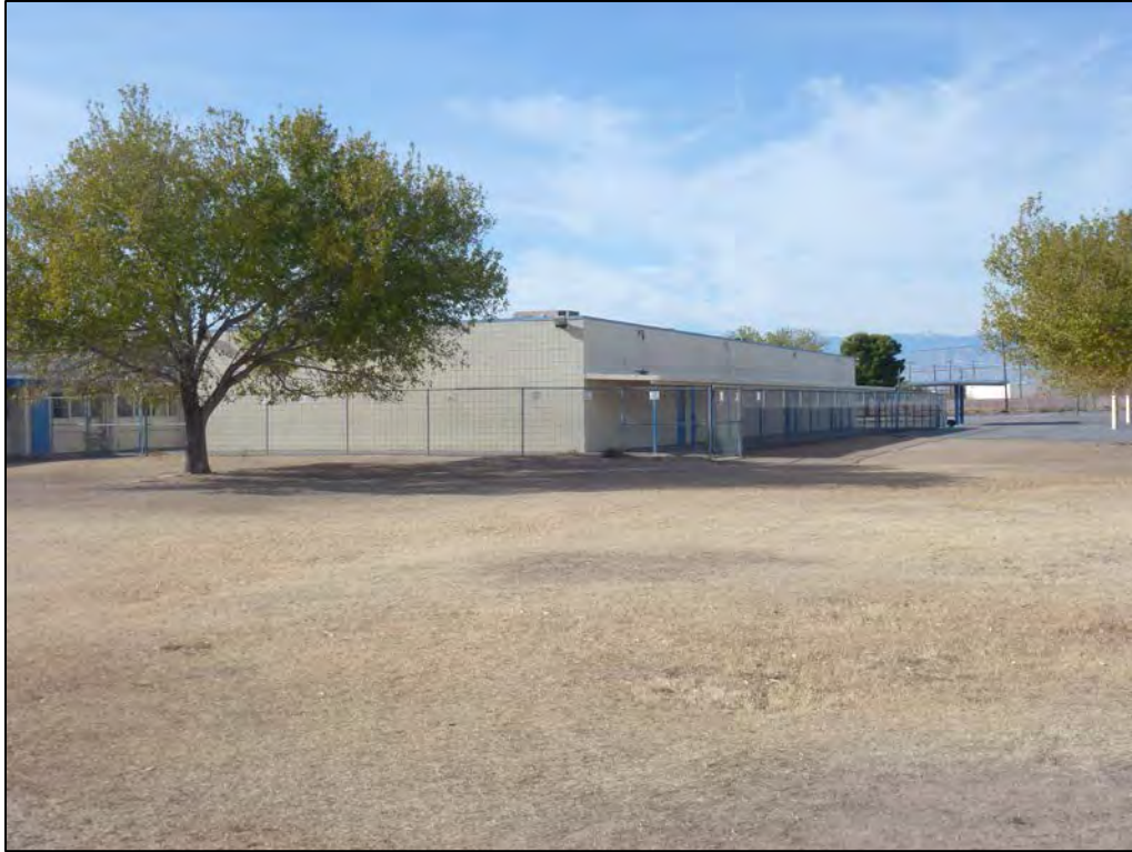
Figure 74. Facility 1787 east and north elevations, looking southwest.
