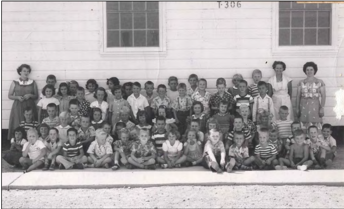
Figure 7. Photograph of the barrack building (T-306), which was used as a classroom, with the students and the teachers. Courtesy of NSM, Lomie G. Heard Collection.
