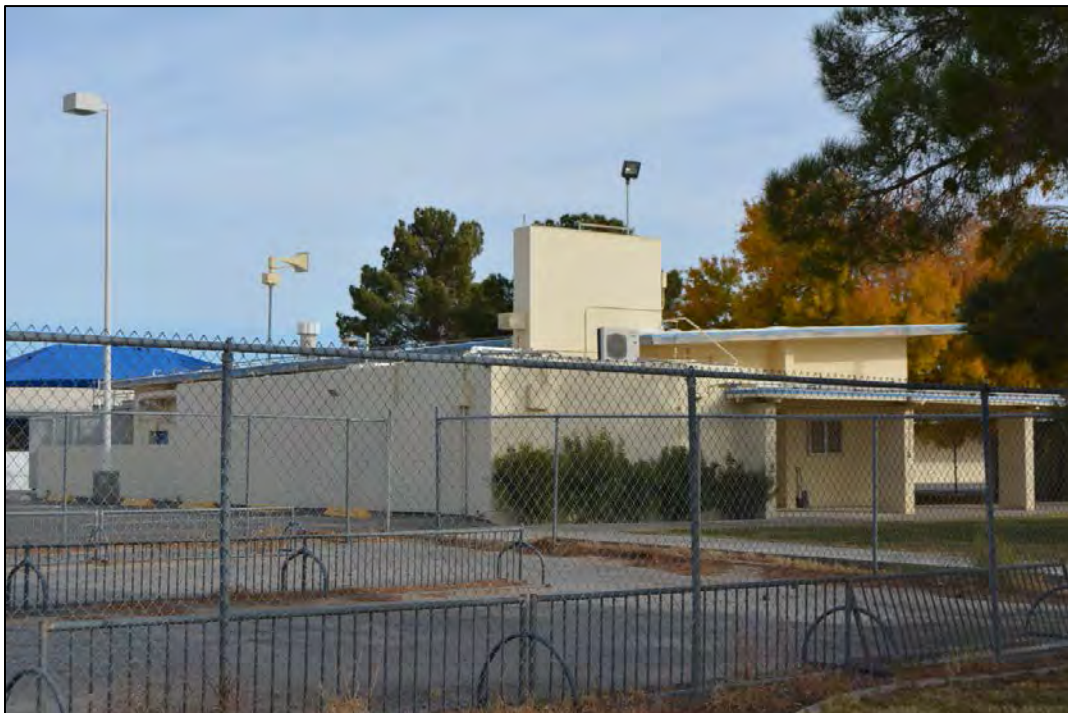
Figure 94. Facility 1790 south and east elevations, looking northeast. Note: Facility 50000 (bicycle rack) is seen in the foreground.
