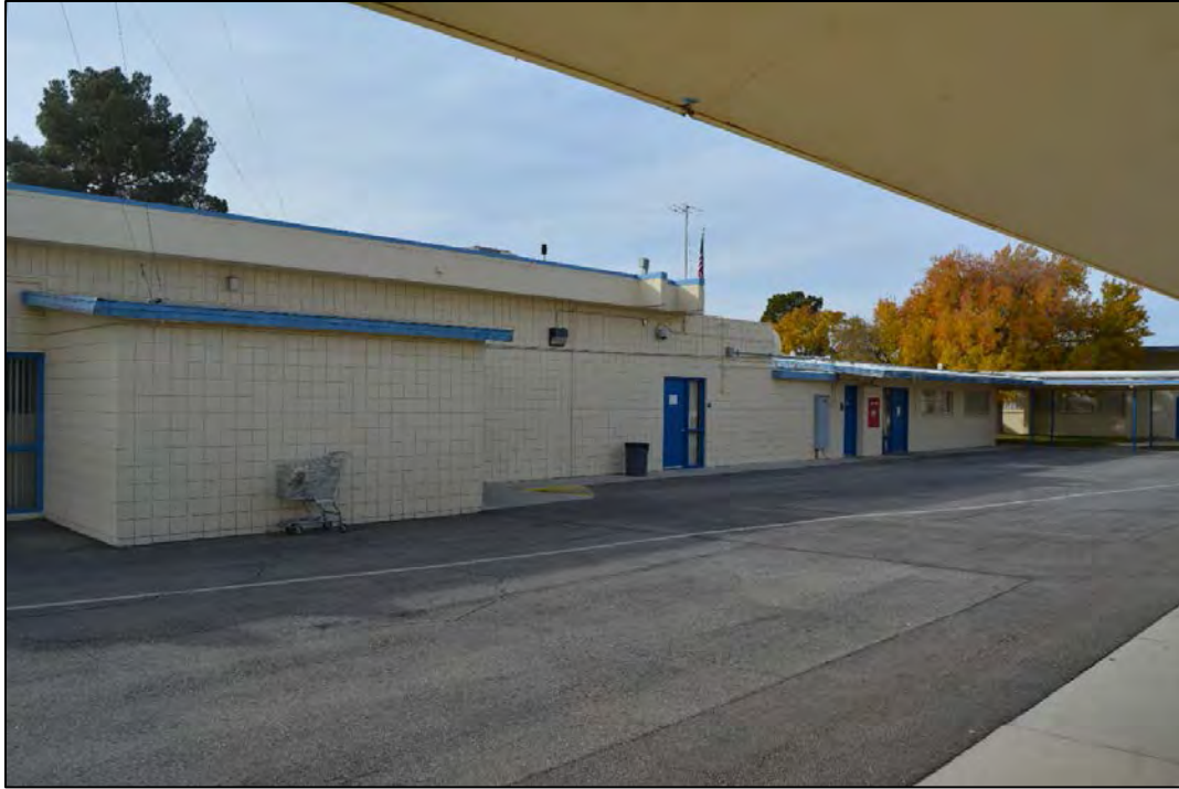
Figure 41. Facility 1781 north elevation, looking southwest.
