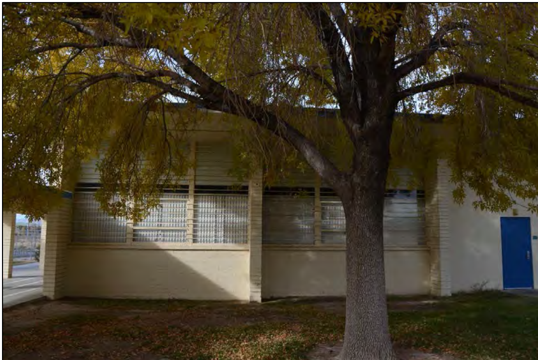
Figure 90. Facility 1790 east elevation, looking west.
