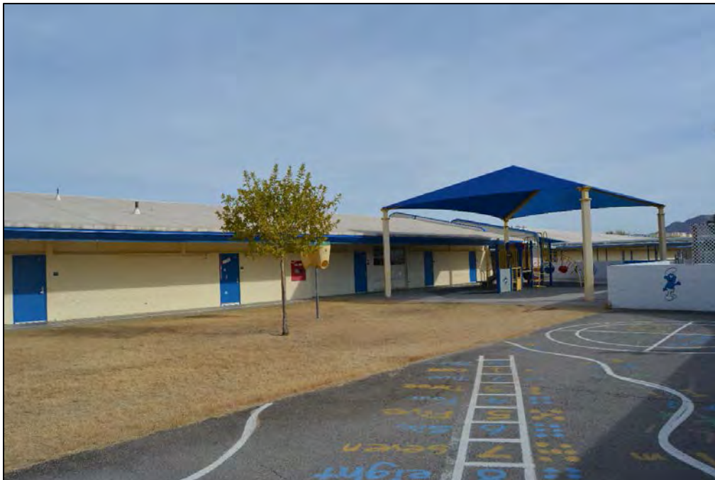
Figure 106. Overhead protection located in the kindergarten playground, looking northeast. Facility 1789 on the left.
