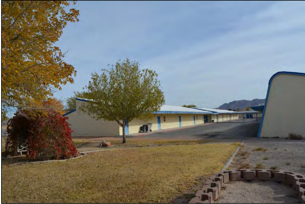
Figure 81. Facility 1788 (left) west and south elevations, looking east, aligned with Facility 1785. Facility 1789 is seen on the right. The school garden is seen on the foreground.
