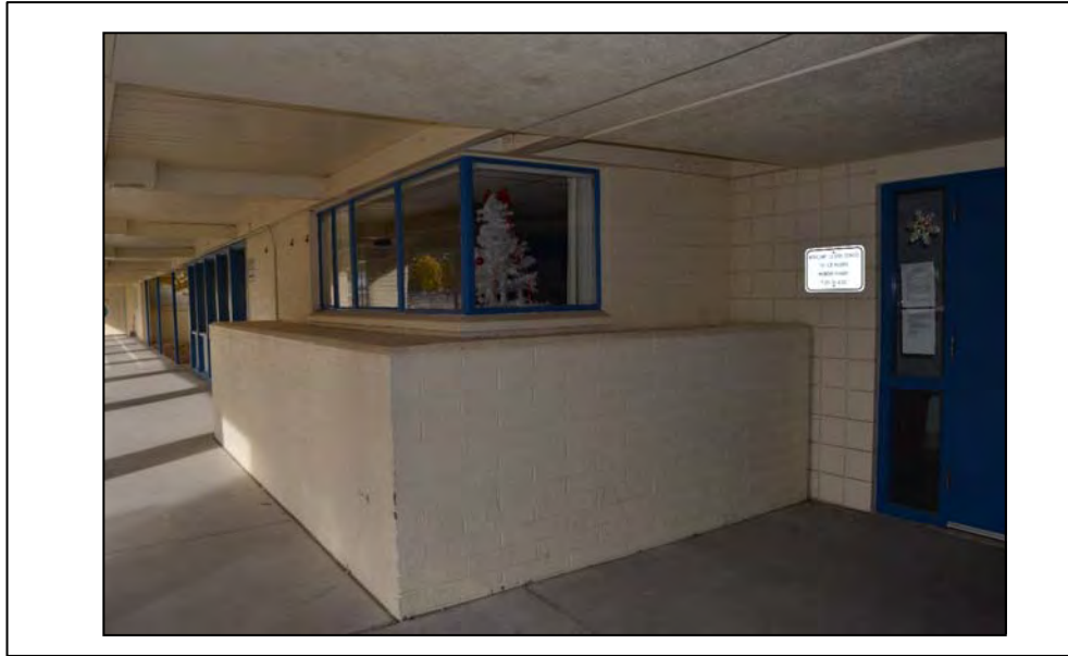
Façade: South Facing: NW Photographer: Serra Akboy-İlk Date: 12/11/16
