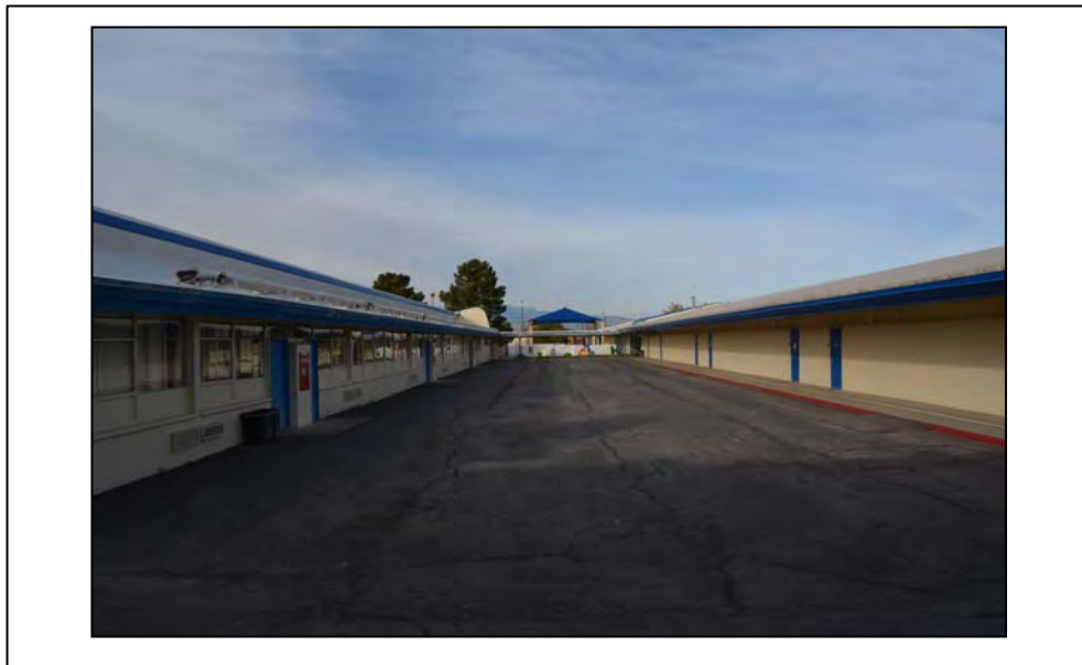
Façade: Courtyard between Facility 1783 (left) and Facility 1784 (right) Facing: W Photographer: Serra Akboy-İlk Date: 12/11/16
