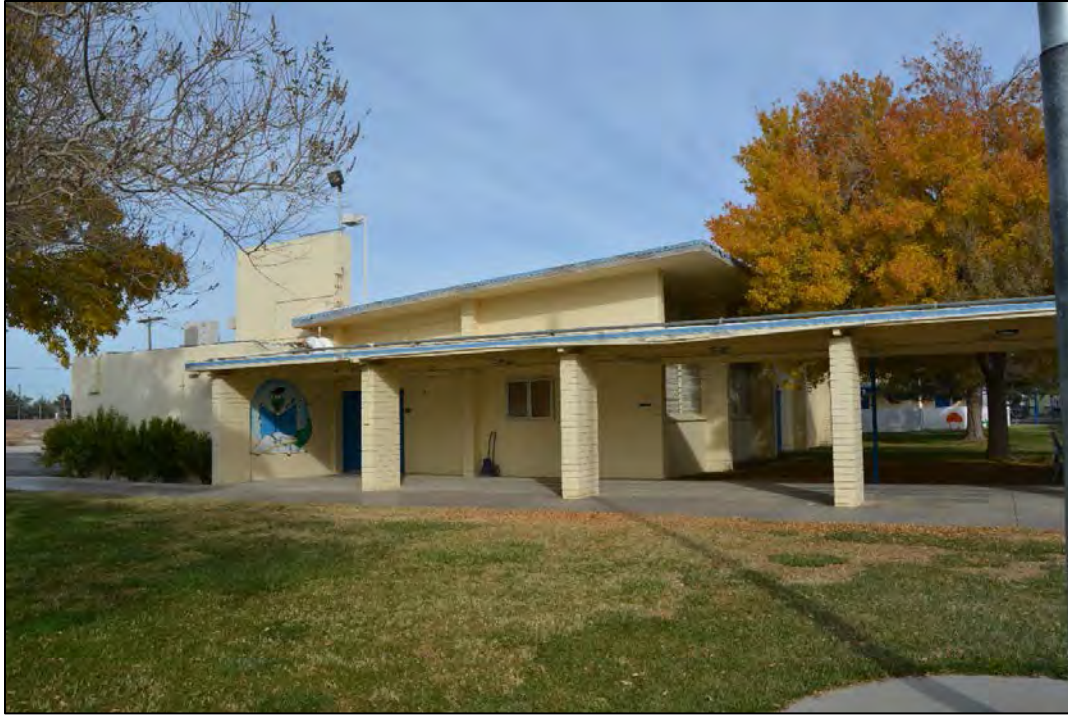
Figure 89. Facility 1790 south elevation, looking north.
