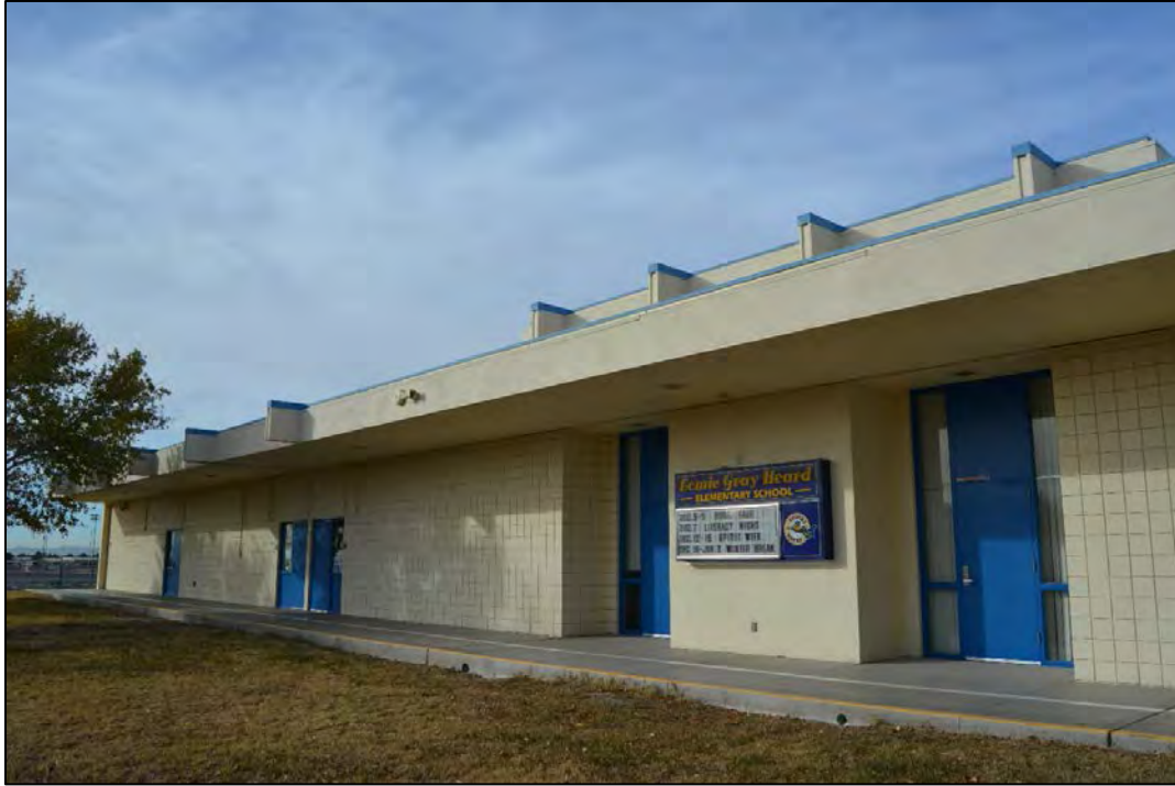
Figure 69. Facility 1786 east elevation, looking southwest.
