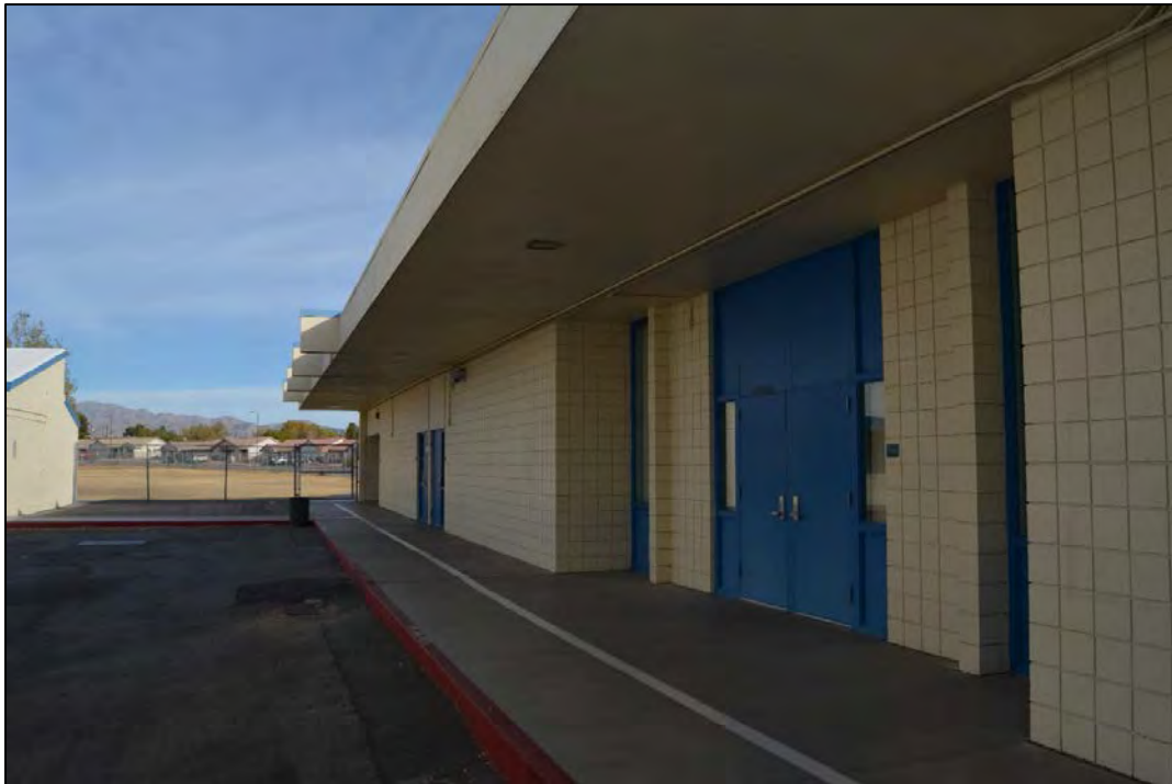
Figure 70. Facility 1786 west elevation, looking north.
