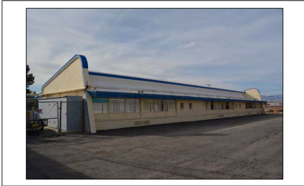
Façade: East & North Facing: SW Photographer: Serra Akboy-İlk Date: 12/11/16
