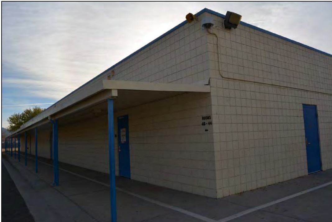
Figure 73. Facility 1787 north elevation, looking southeast.
