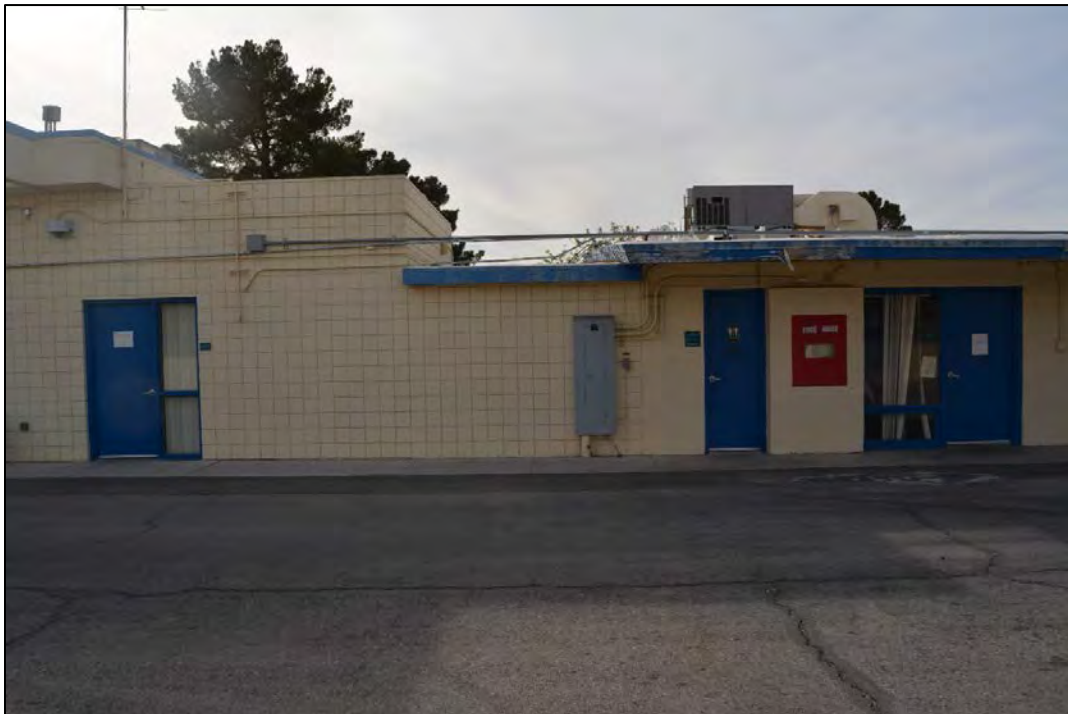
Figure 42. Facility 1781 north elevation, looking south. Note: The change in the structural qualities of the 1953 building (left) and the 1967 addition (right) are evident from the elevations.
