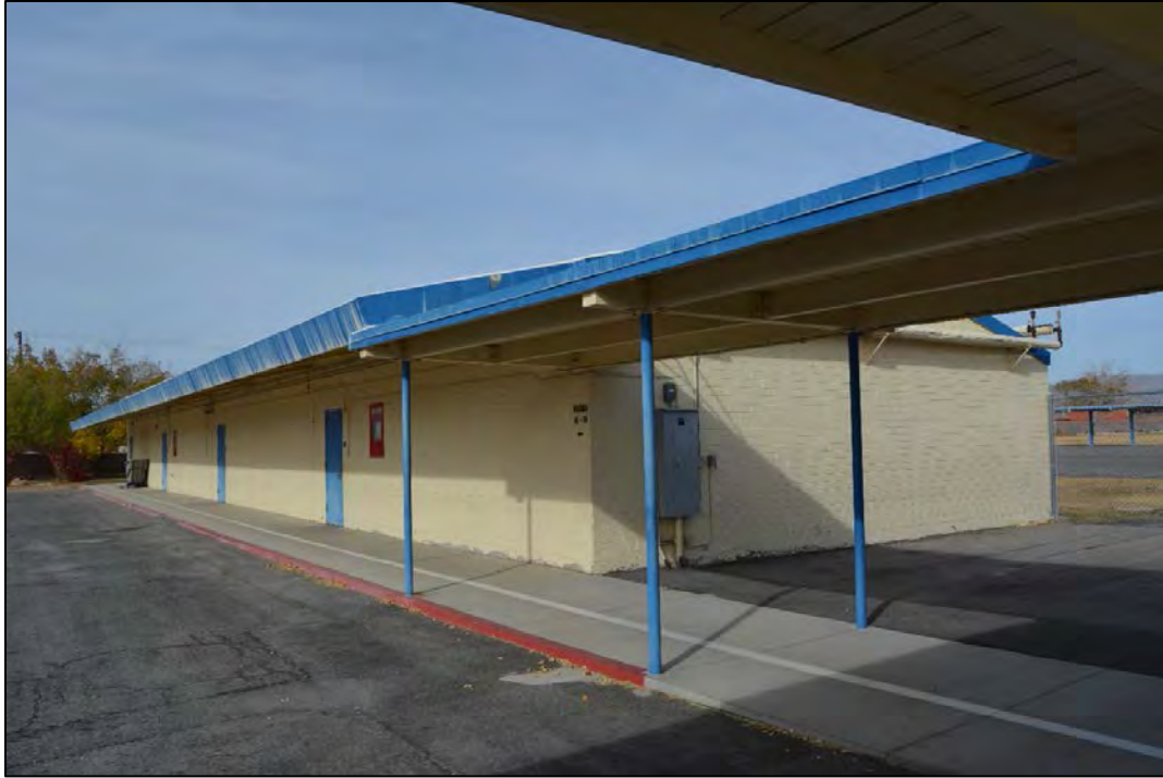
Figure 79. Facility 1788 south elevation, looking northwest.
