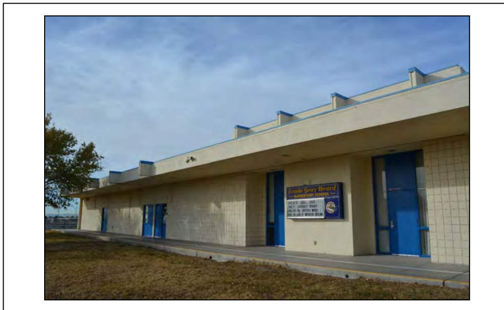
Façade: East Facing: SW Photographer: Serra Akboy-İlk Date: 12/11/16
