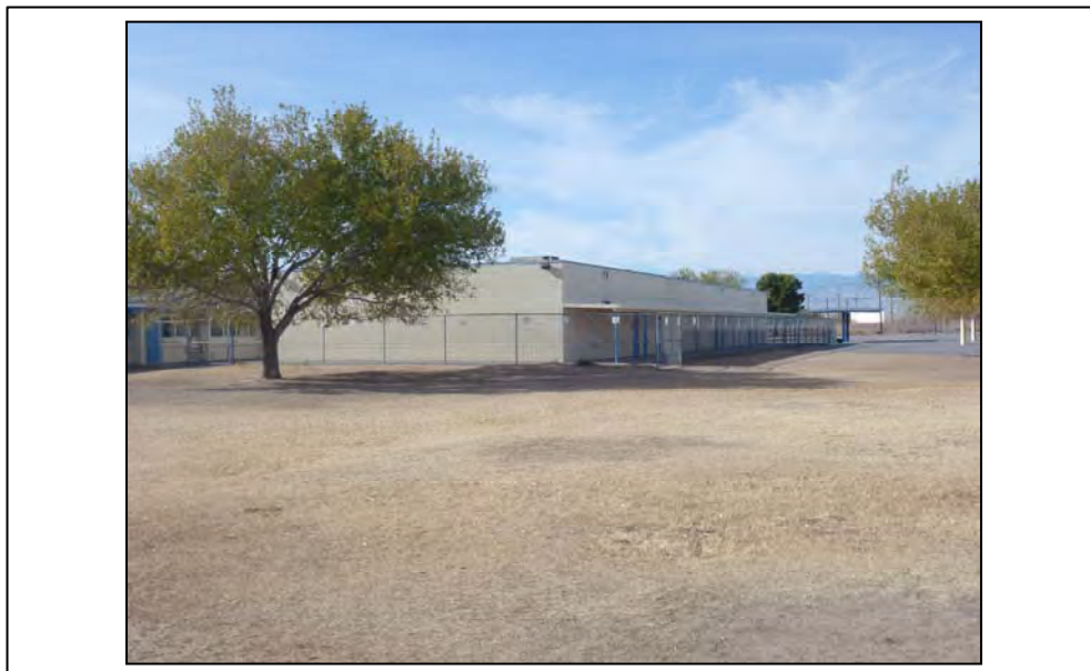
Façade: East & North Facing: SW Photographer: Michelle Wurtz Date: 12/11/16
