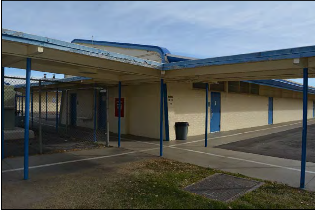
Figure 58. Facility 1784 west and south elevations, looking northeast.
