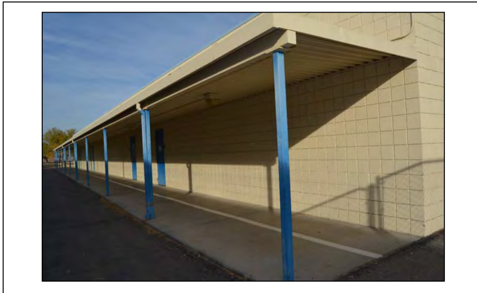
Façade: North Facing: NW Photographer: Serra Akboy-İlk Date: 12/11/16
