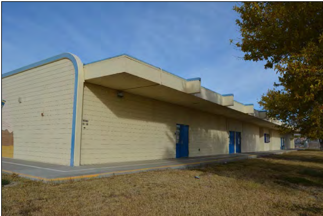
Figure 68. Facility 1786 east elevation, looking west.
