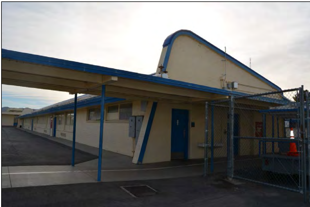
Figure 57. Facility 1784 west and north elevations, looking southeast.
