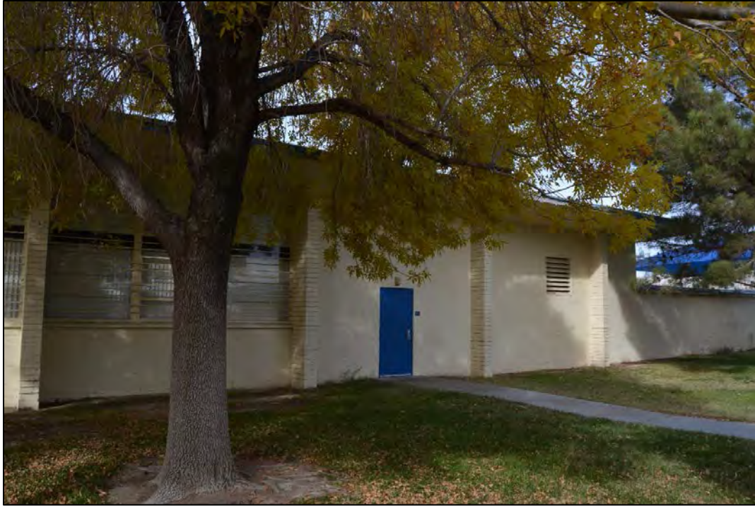
Figure 91. Facility 1790 east elevation, looking west.
