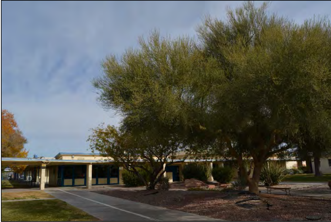
Figure 111. Sidewalk in front of Facility 1781, looking north.
