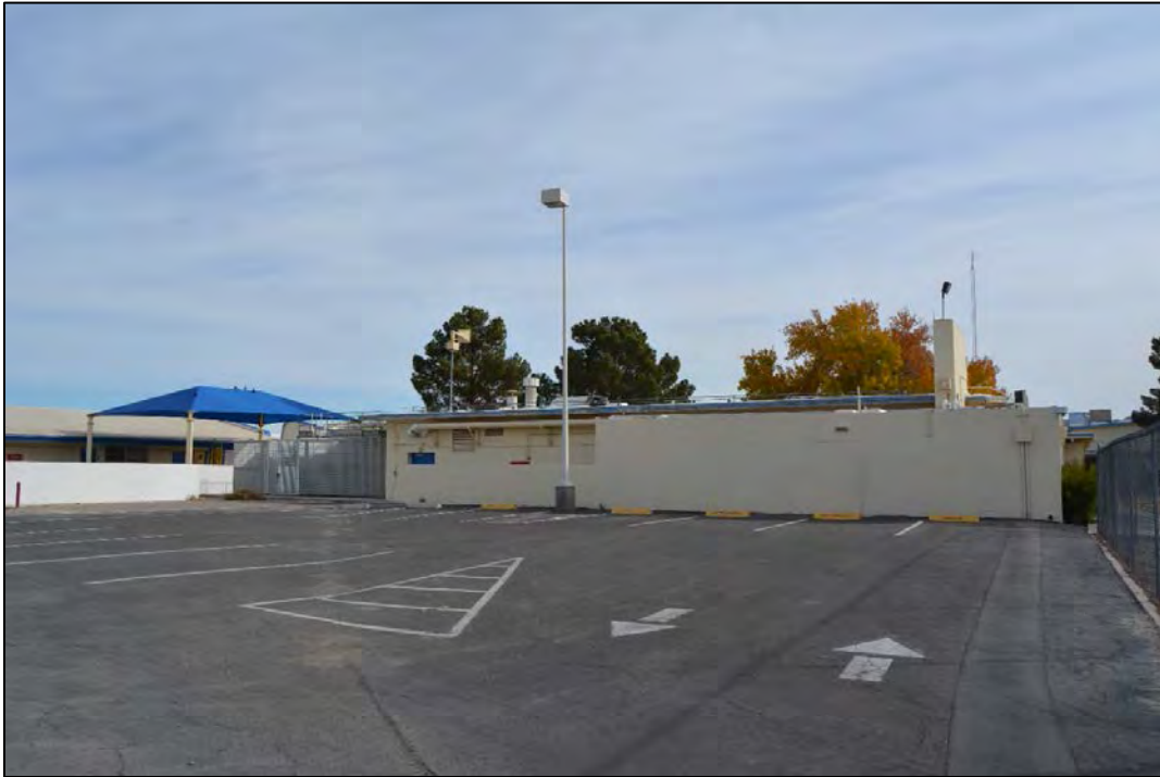
Figure 107. Parking located west of Facility 1790.
