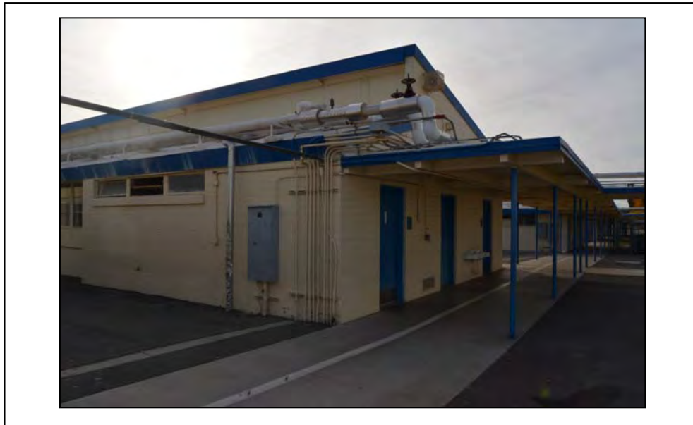
Façade: West and North Facing: NE Photographer: Serra Akboy-İlk Date: 12/11/16
