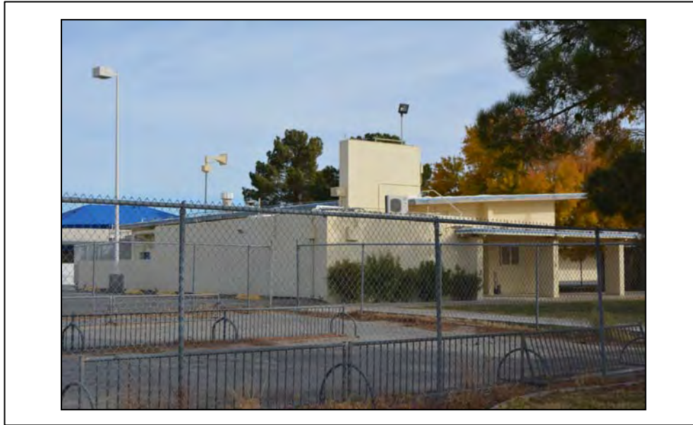
Façade: South & East Facing: NE Photographer: Serra Akboy-İlk Date: 12/11/16
