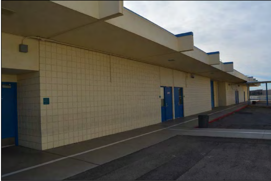
Figure 71. Facility 1786 west elevation, looking south.
