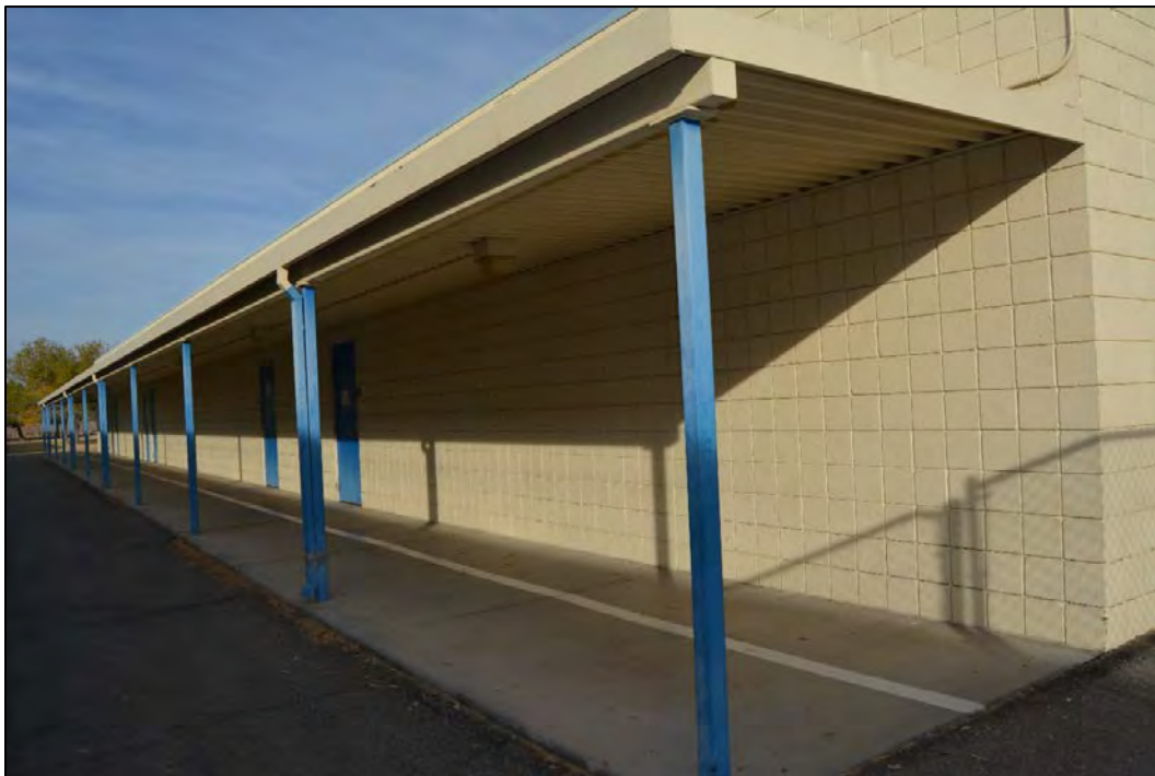
Figure 75. Facility 1787 north elevation, looking northwest.
