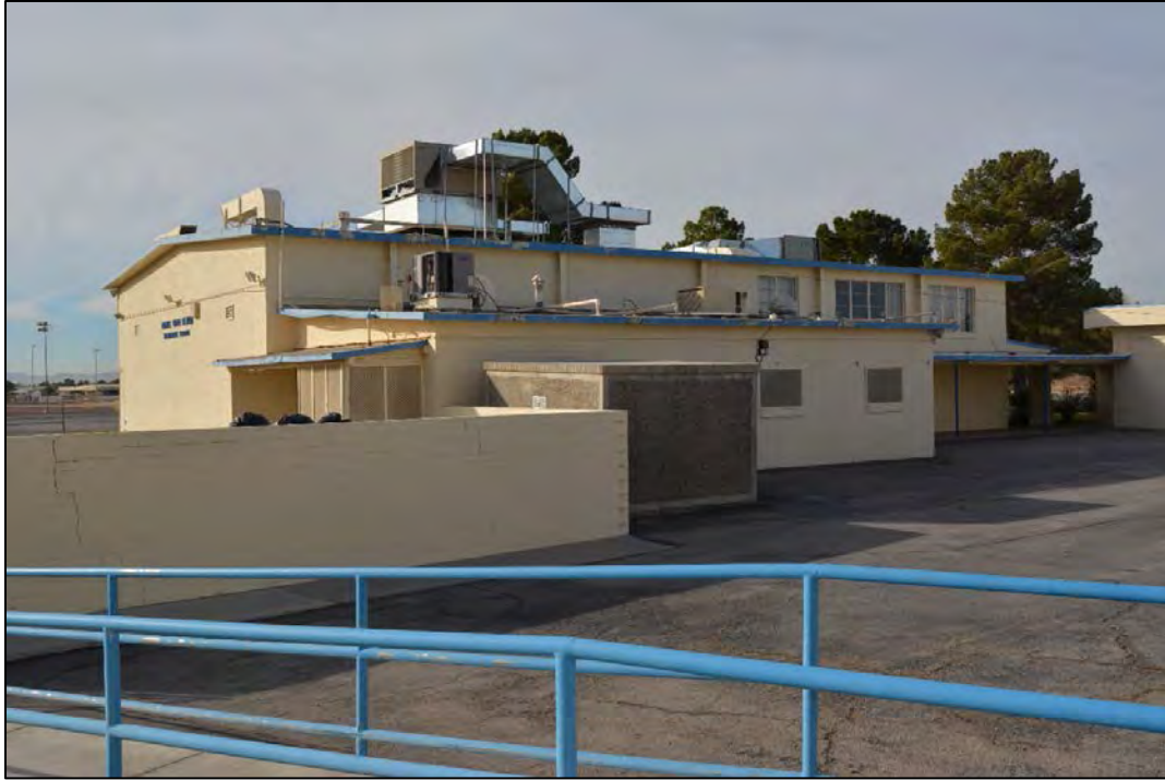
Figure 47. Facility 1782 east and north elevations, looking southwest.
