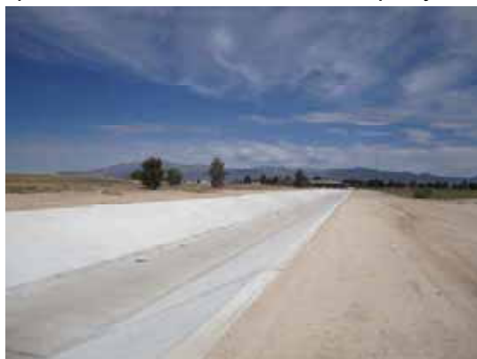
Photograph 3-2. Sloan Channel which bisects the proposed project site.
